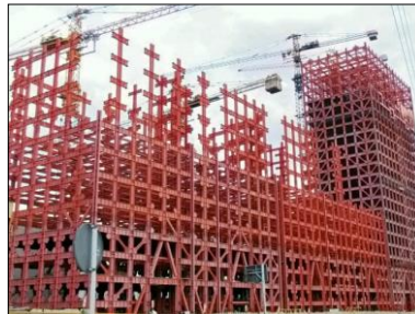
Figure 3. Steel frame system in Iran
