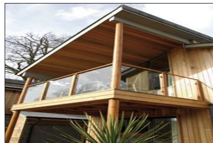
Figure 2. Prefabricated wood frame building
