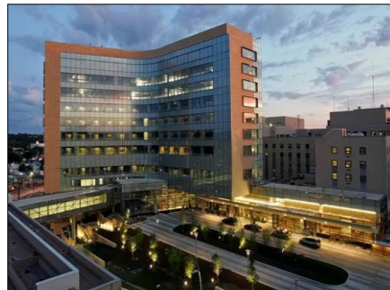
Figure 1. The prefabricated building
